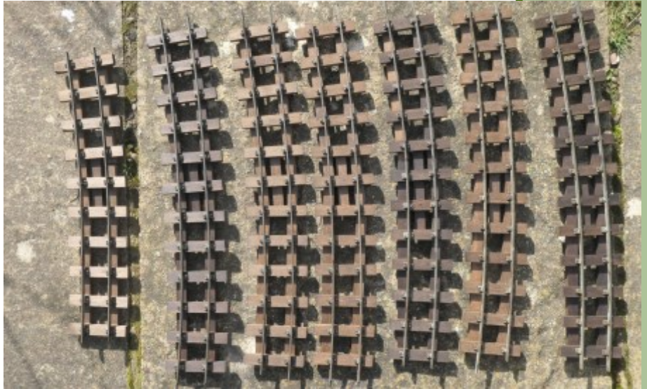
Photo 5 Rebuilt creosoted track ready to lay.
