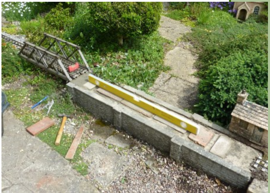
Photo 6 Brick pavers replacing the timber base in the embankment.
