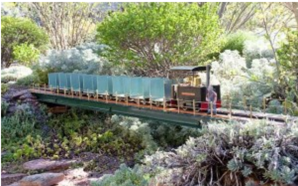
Photo 4 Single-span bedrails, sporting added handrails, form the present-day east bridge.
