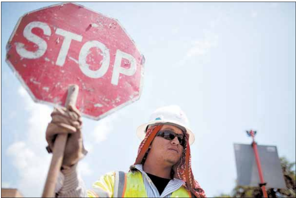
Construction worker Jose Lopez redirects traffic at Dean Keeton Street and Whitis Avenue while construction blocks lanes on both streets to improve a water line that runs beneath the University.
