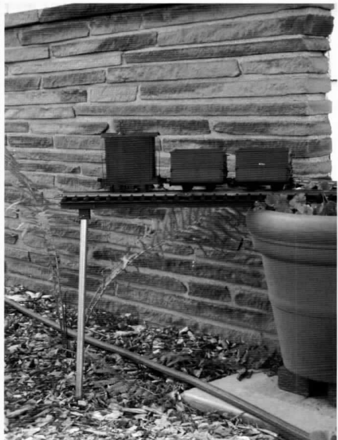
Below: This shot demonstrates the method used to support the railbed sections. (No, not the flower-pot!)
