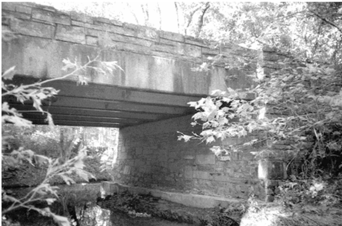
Limestone Creek Bridge, circa 1999. (CNRA archives, LCS photograph).
