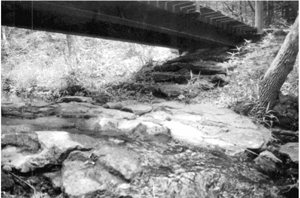
Stone low water crossing leading from north parking area to Travertine Island, with bridge above, date unknown.
