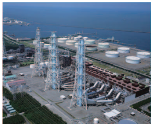
Fig. 3 Higashi-Niigata Thermal Power Station
