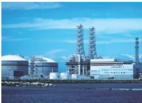
Fig. 8 Shin-Sendai Thermal Power Station
