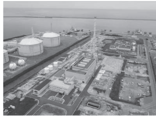
Fig. 9 Joetsu Thermal Power Station
