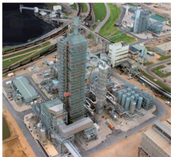
Fig. 14 Panoramic view of a modern commercial CCS plant (9)
