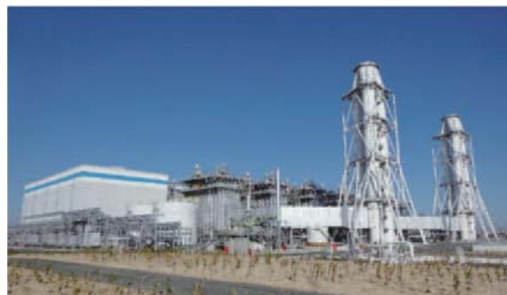
Fig. 11 Nishi-Nagoya power station block no.7-1 and 7-2
