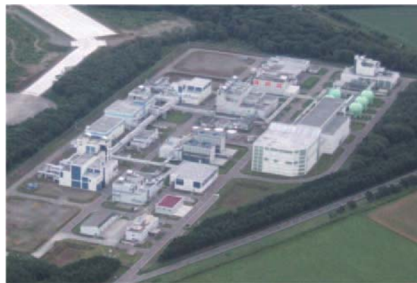
Fig. 1 Overview of CTC (Chitose test center aero-dynamics & propulsion test facility)
