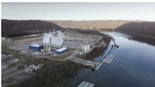
Fig. 17 Hydrogen blending demonstration at Long Ridge combined cycle power plant (Photo by GE Gas Power)
