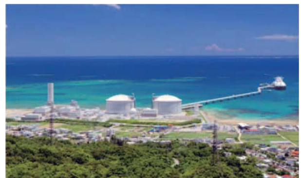
Fig. 11 Overview of Yoshinoura Thermal Power Plant
