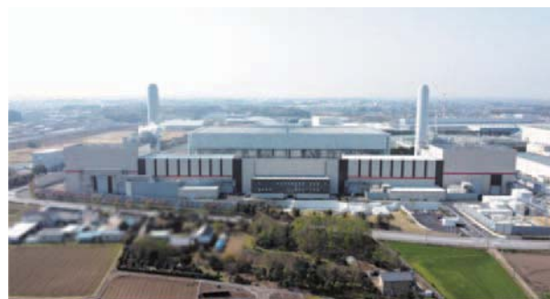
Fig. 12 Overview of Moka Power Plant
