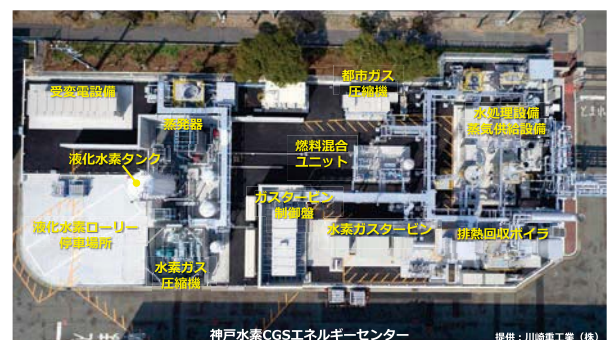
Fig. 5 Kobe hydrogen cogeneration panoramic view
