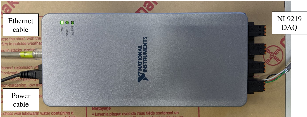
Figure 24. NI 9181 chassis with attached NI 9219 DAQ unit
