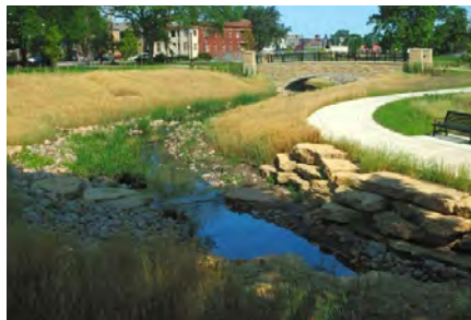
Stormwater bio-retention areas designed into attractive park features such as a stream
