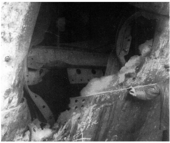
Figure 6: A close-up of the damage to the *RMS Olympic* due to collision with the *HMS Hawke* in the Solient in 1911. Note the man for scale. A considerable amount of plasticity in the hull plates is indicated by the bending and twisting seen in the picture. Note missing rivets. Photo from [25].
