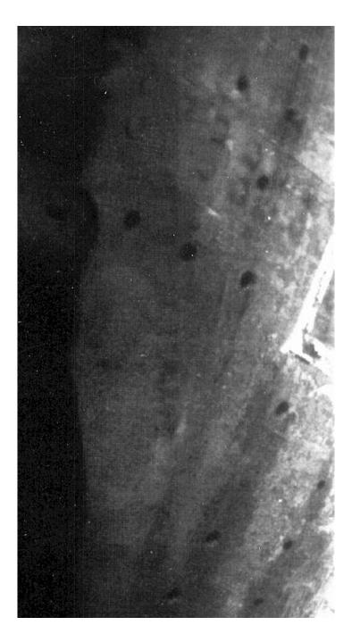
Figure 8: Blowup of damage to *Olympic* after collision with *HMS Hawke*. This image has undergone a considerable amount of digital image processing to bring out the empty rivet holes. On the entire image after processing, one can identify in excess of 50 rivets missing from the immediate area of the impact. Image from [25].
