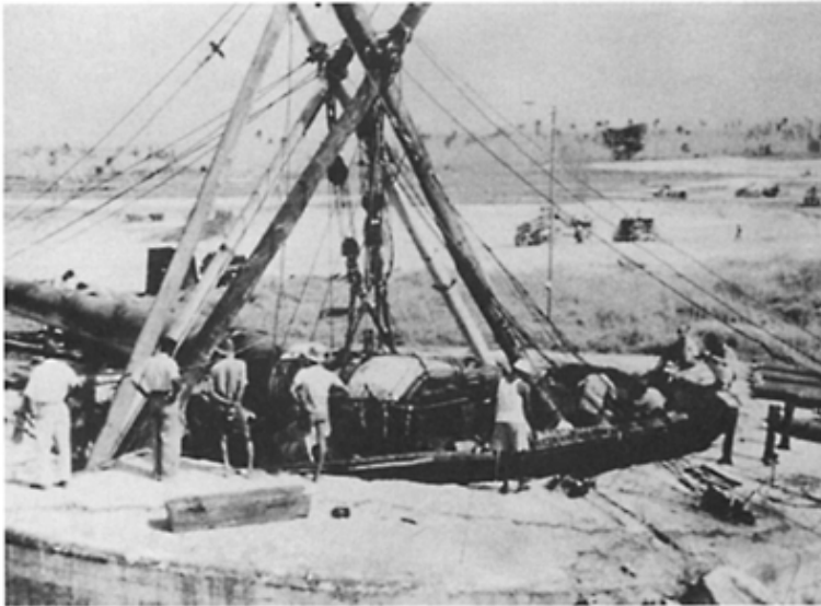
Plate 5.9 Local contractors removing one of the biggest guns with a crude wooden structure in 1948. It was destined for the UK, for use as scrap.
