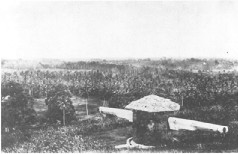
Plate 3.7 A rangefinder badly disguised as a local attap hut.
