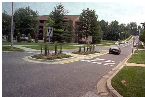
Center planted medians encourage drivers to slow down. Breaks in roadway provide safer crossings for pedestrians.
