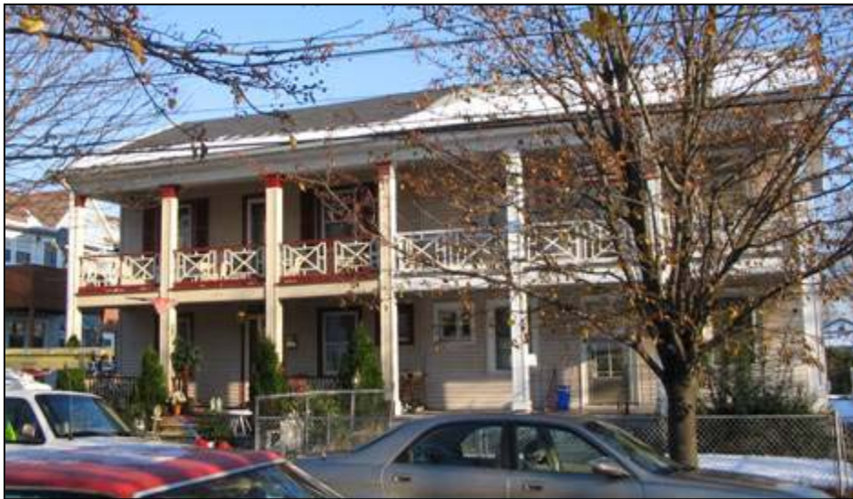
Historically Sympathetic Restoration
