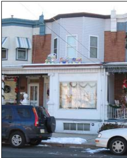
Historically Unsympathetic Restoration
