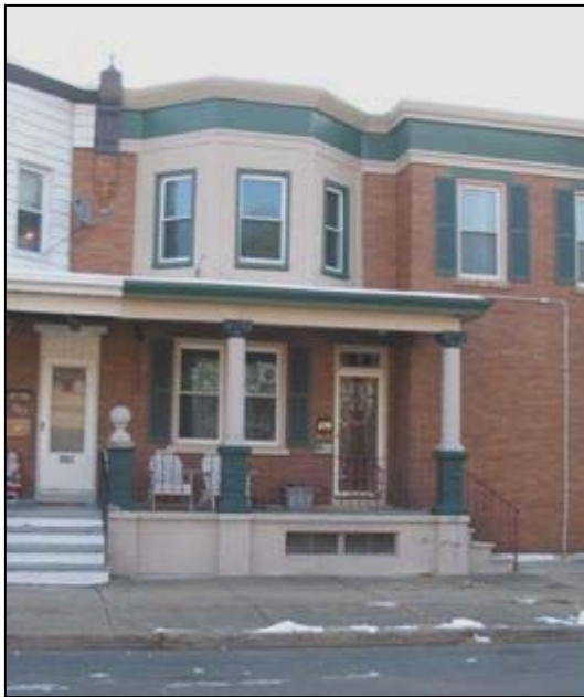
Historically Sympathetic Restoration
