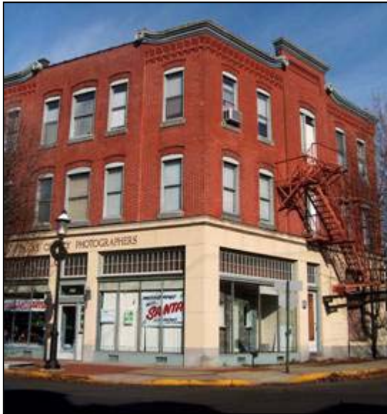
Historically Sympathetic Restoration
