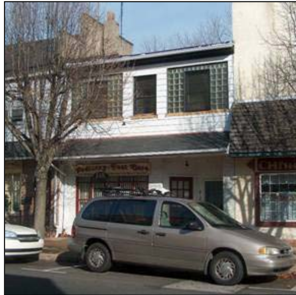
Historically Unsympathetic Restoration
