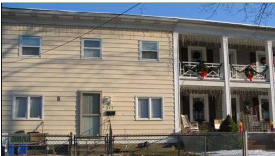
Historically Unsympathetic Restoration
