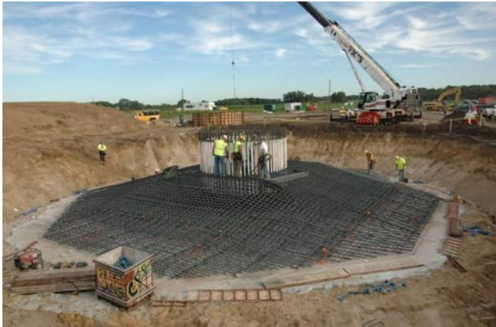
Figure 3.10 A Typical Turbine Foundation being Constructed
