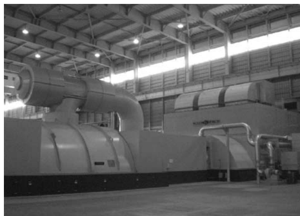
Figure 9 Group 4 stage 4-1 power train (GT & ST)
