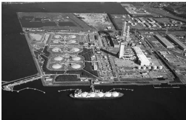
Figure 1 TEPCO Futtsu thermal power station
