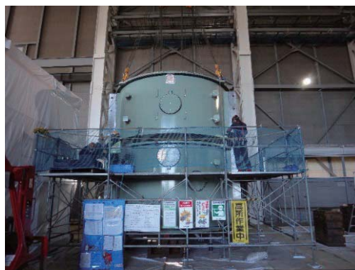
Fig. 11 Stator frame assembly
