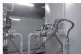
Gas emergency shutoff valve
