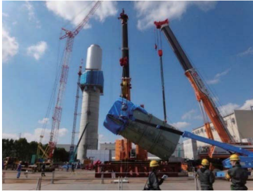
Fig. 12 Overturn stator frame by two cranes
