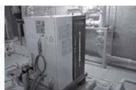
Air compressor for instrument
