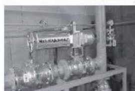
Gas emergency release valve
