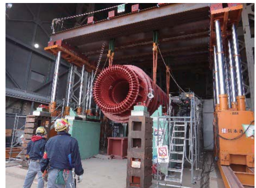
Fig. 15 Stator hoisting by PJS
