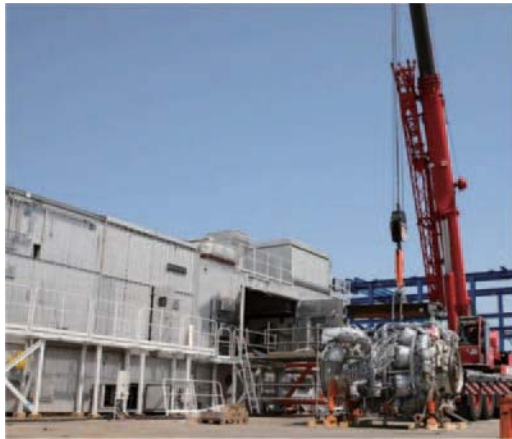
Fig. 6 SGT-750 core engine exchange (off-shore application)
