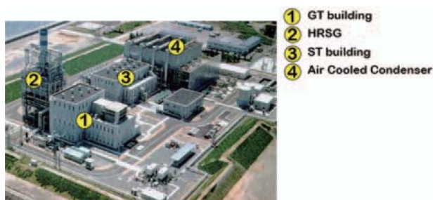
Fig. 3 Gas turbine combined cycle power plant (Validation facility) in takasago factory
