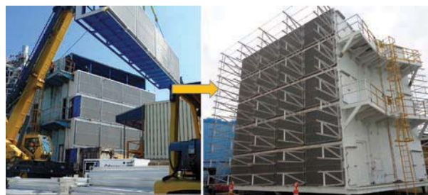
Fig. 15 Rehabilitation of GT intake filter house
