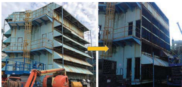
Fig. 14 Rehabilitation of GT intake filter house
