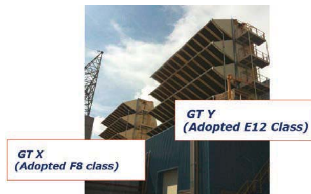
Fig. 1 GT intake filter house
