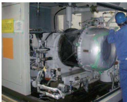
Fig. 8 Private power generator (twin)
