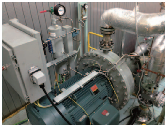
Fig.13 General View of 200kW VPT on The Test Engine
