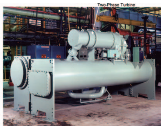
Fig. 5 Carrier 19 XRT Chiller with Two-Phase Turbine
