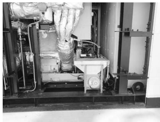
Fig. 13 MGT installed in SOFC
