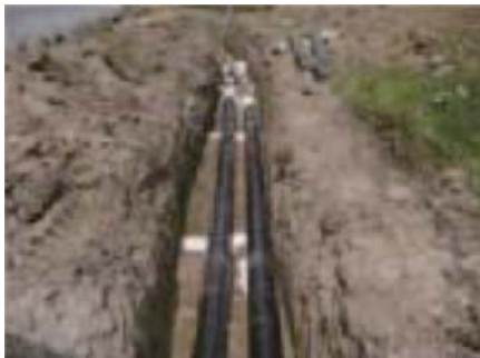
Fig. 10 Hot water piping distribution
