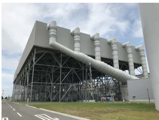
Fig. 7 Landscape of Air-Cooled Condenser (ACC)
