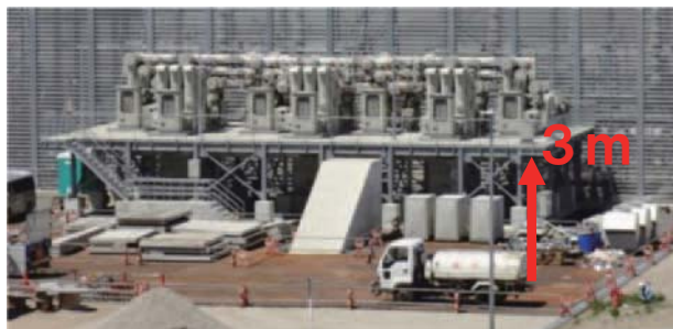
Fig. 8 Outdoor switchyard raised by 3m above the ground
