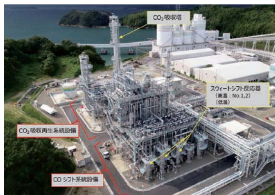
Fig. 11 CO 2 capture unit
