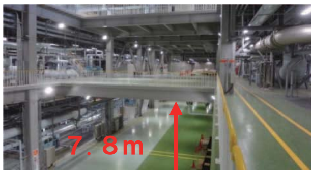
Fig. 7 Important install equipment such as electrical equipment on the second floor and above
