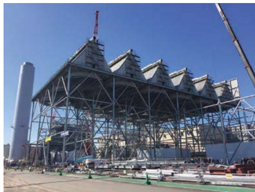
Fig. 8 No.1 ACC under construction
