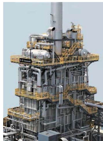
Fig. 6 Heat Recovery Steam Generator
