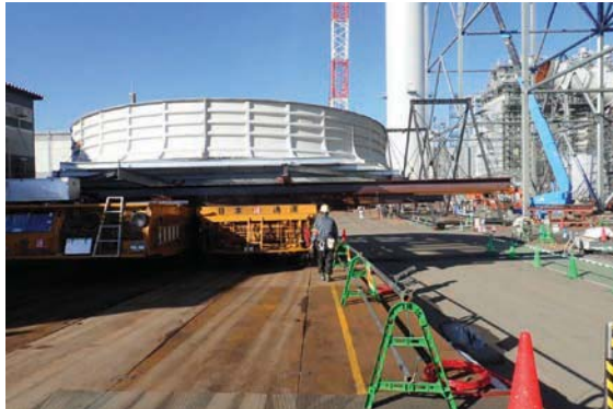
Fig. 16 Transport of assembled equipment in construction area (ACC Fan Ring)
