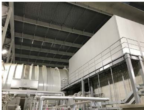
Fig. 6 Inside-scape of No.1 steam turbine building 「Exhaust steam duct (left side), Generator case (right side)」
