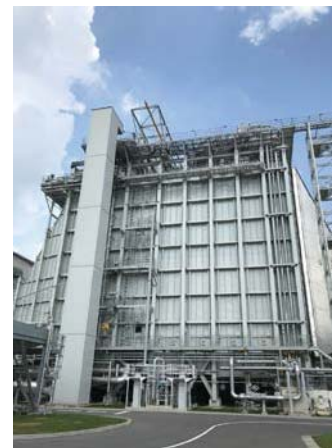
Fig. 5 Heat recovery steam generator
