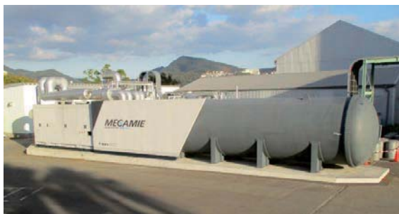
Fig. 14 MW class SOFC half module (Provided by Mitsubishi Power, Ltd.)
