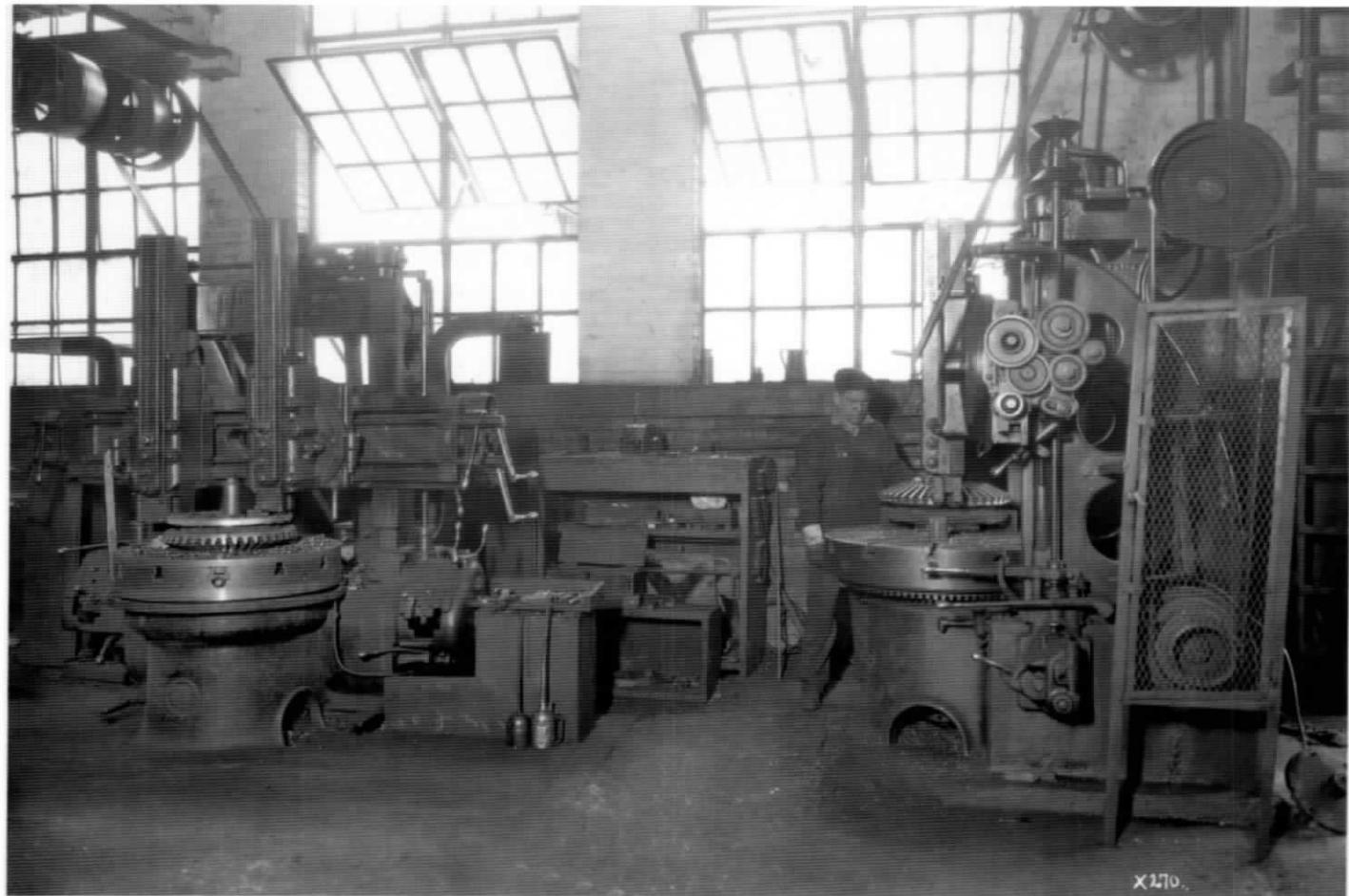
Photo 1. Shay bevel gear production. Courtesy of the Allen County (Ohio) Historical Society
