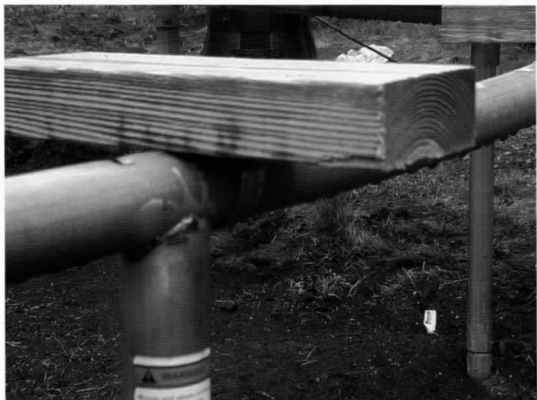
A subroadbed joist is shown mounted to a curved section of the frame, prior to the positioning and mounting of the Trex subroadbed sections.
