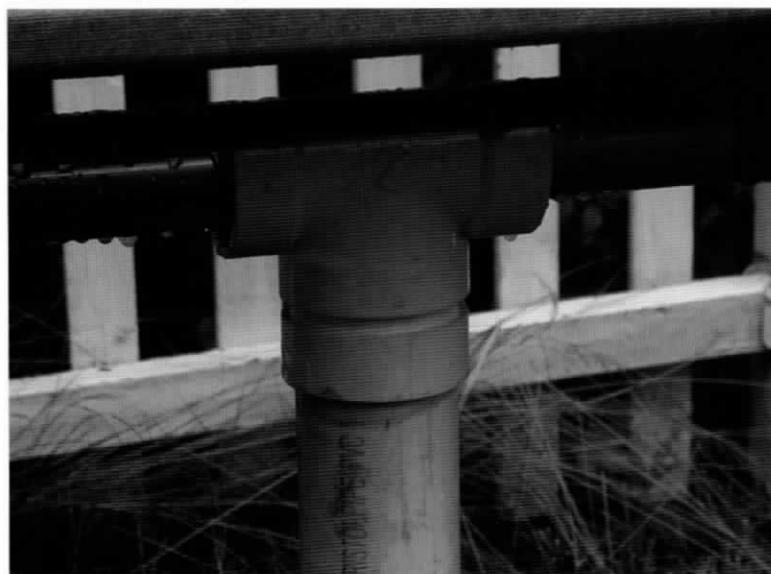
This photo shows a Waste Tee "Saddle" supporting the electrical conduit portion of the frame.
