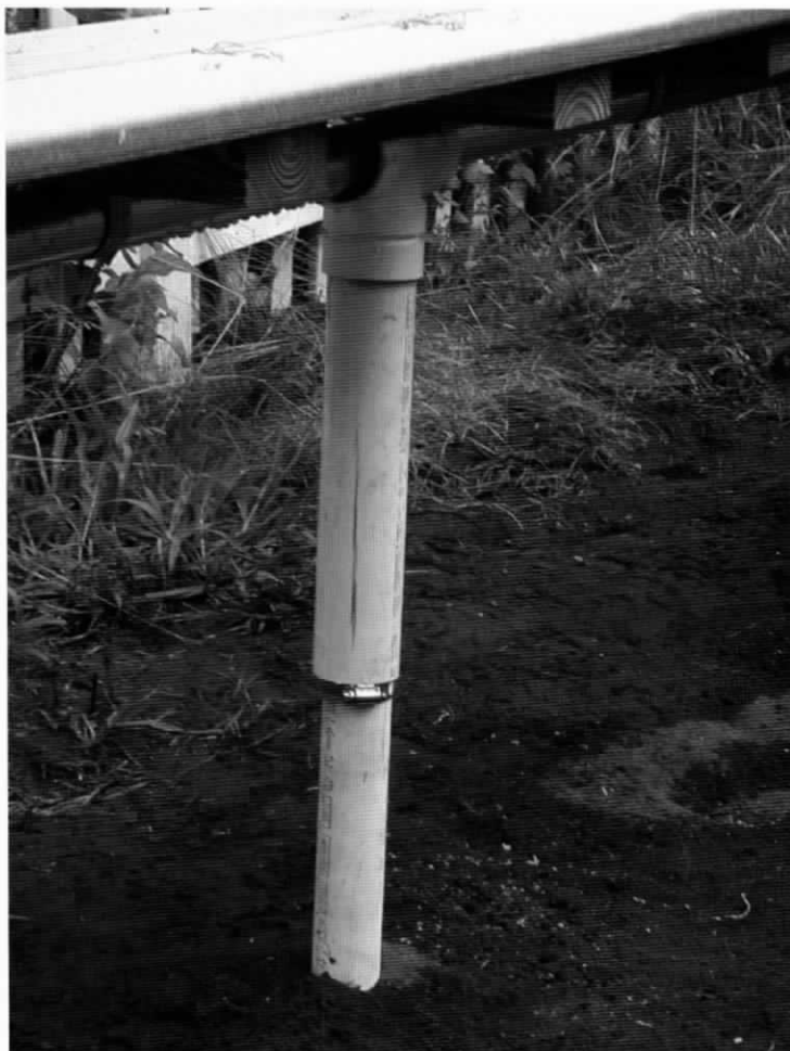
The adjustable PVC leg sections are leveled and held in place by the band clamp shown just below the 2" PVC top leg section.
