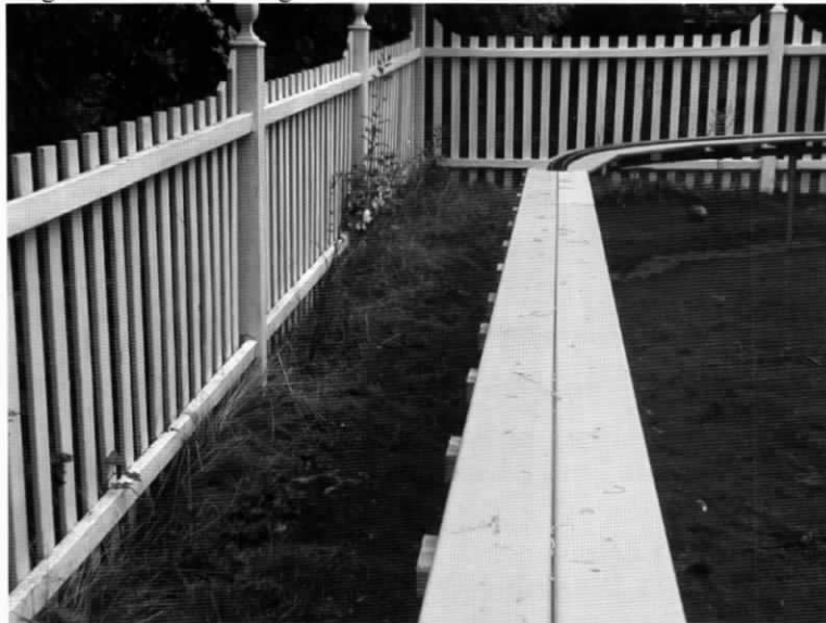
Track laying began with the two curved end sections, followed by the back and front straight sections. The seams between the Trex boards allow for runoff of water and snow, as this railroad performs equally well year round.,
