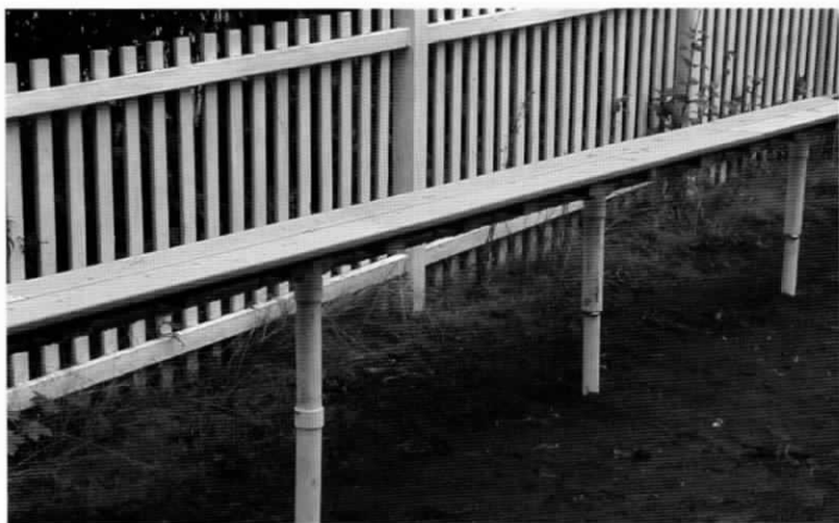
The back straight section of the railroad is all set, leveled and ready to accept track.
