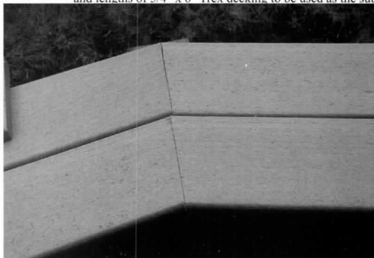
The Trex subroadbed was cut at 22.5 degree mitered angles to form the hexagonal shaped curves for the end frames.
