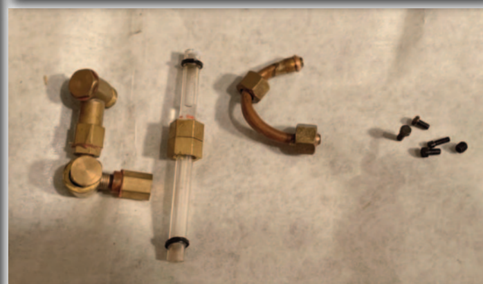
Photo 2 - Sight glass plumbing after a careful removal to avoid breakage. Pieces are laid out on the sticky side of tape to avoid losing anything, plus it holds it in its original alignment.
