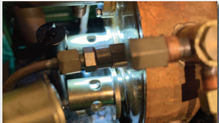
New burners in place, fittings back, ready for a run.
