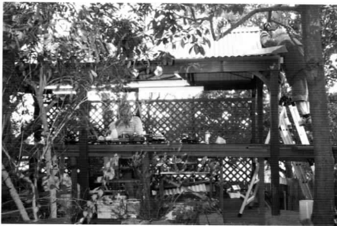
Mark and Laurie finish the flashing on the roof of the nearly completed station.
