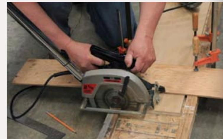
FIGURE 14: cutting the engineered beams to length. Using the vacuum keeps dust generation to a minimum in the train room.
