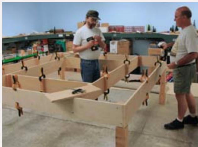
FIGURE 10: Construction of the helix table under-the-surface bracing.
