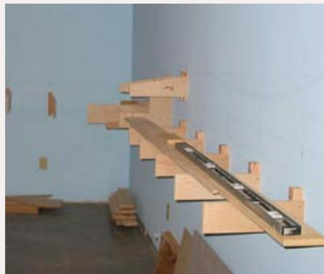
FIGURE 5: More joists and cleats.
