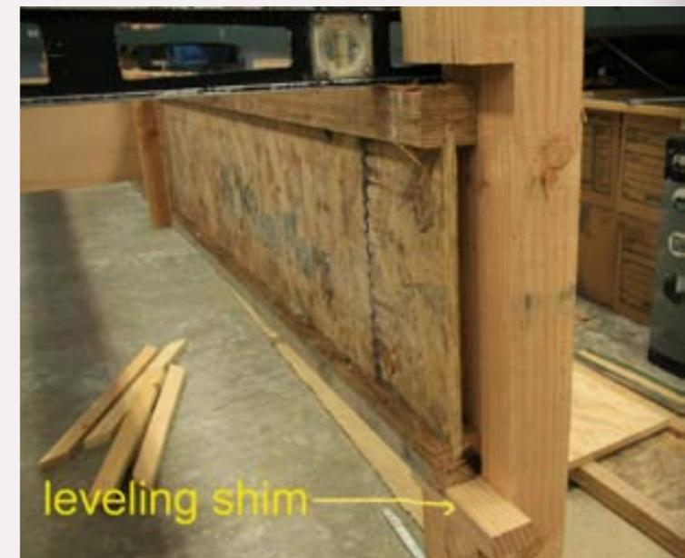
FIGURE 15: Shimming the engineered joists to level them.
