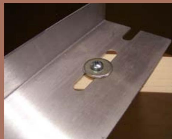
Figure 79: Securing mounting bracket.
