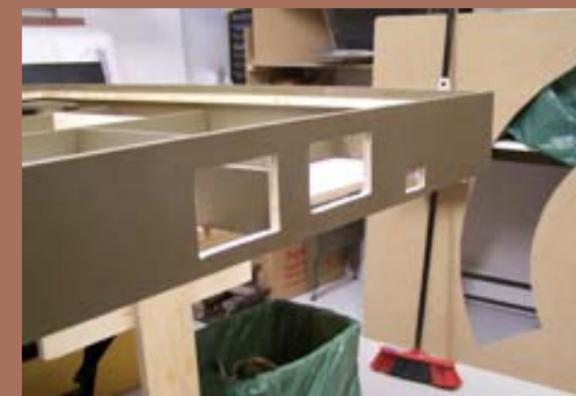
Figure 37: Holes for the fascia-mounted components.
