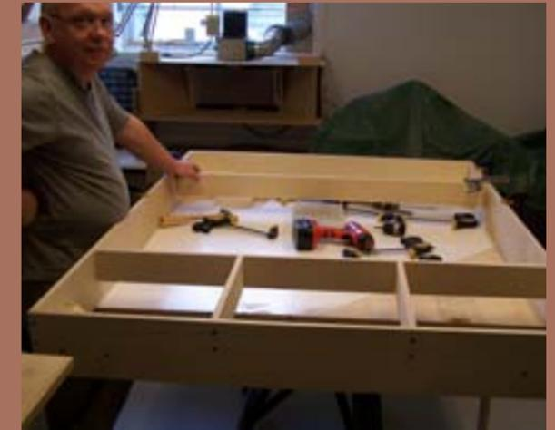
Figure 16: Assembling sideframe and gusset. I couldn't have assembled the module without Ray's help.
