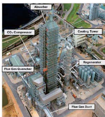
Fig. 13 World's largest CO 2 recovery plant
