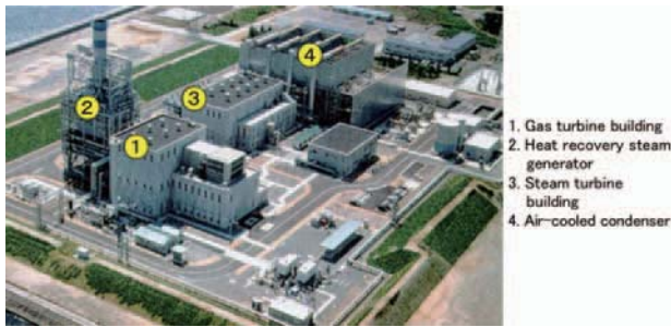
Fig. 3 MHPS takasago works T-point demonstration combined cycle power plant
