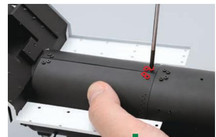
Tighten the four screws removed in Step 4 into the holes in the bottom of the smokebox.
