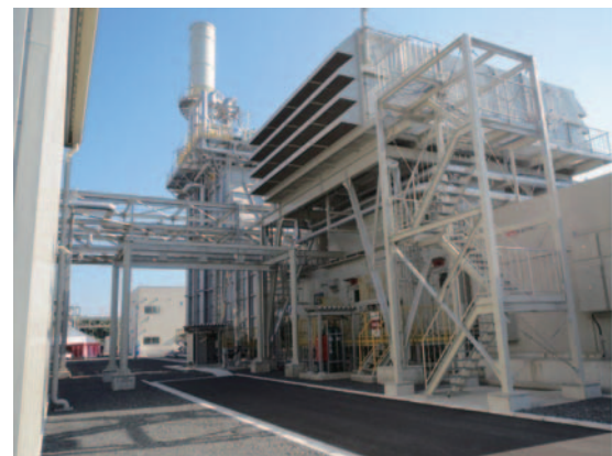
Fig.19 LM6000 package for Shin-Nakasode power plant
