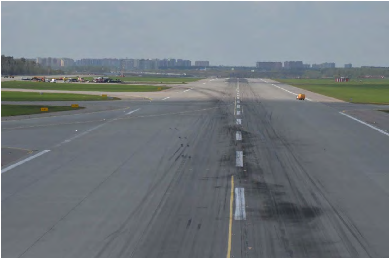
Fig. 38. The onset of the left shift traces off the RWY centerline at the area of the A5 TWY
