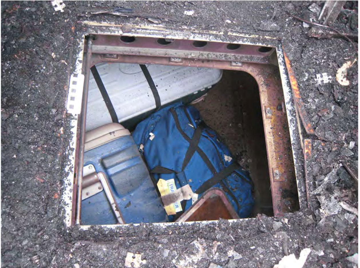
Fig. 19. External view of the rear baggage compartment after the accident
