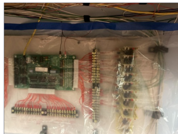
4. I used plastic dropcloths to protect the electronics for signals from water drips.
