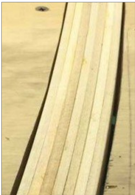
11. Solid spline sub-roadbed.
