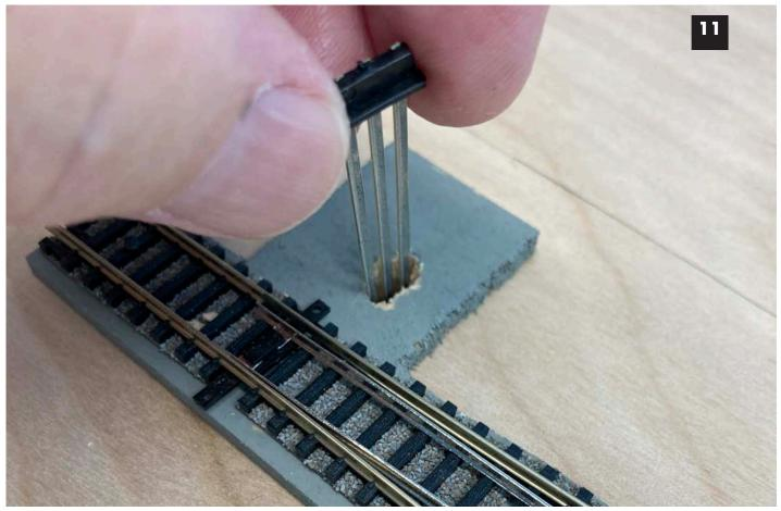
$\label{lem:lemage 11.} \textbf{Image 11.} \ \textbf{Test fit the wiring connector and keep sawing until it fits.}$
