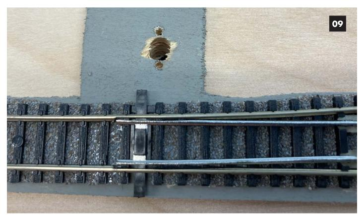
**Image 09.** Next a larger center hole is drilled. I use a 7/32" drill.
