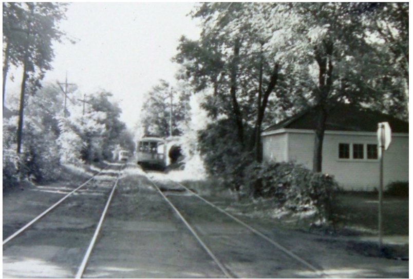
On one section of the Twin City Line, the right of way was down an alley behind the homes. This was a distinguishing feature the Forrest wanted to model.
