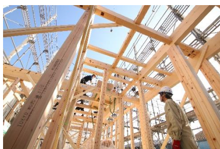
Construction of a house using TOKYO WOOD
