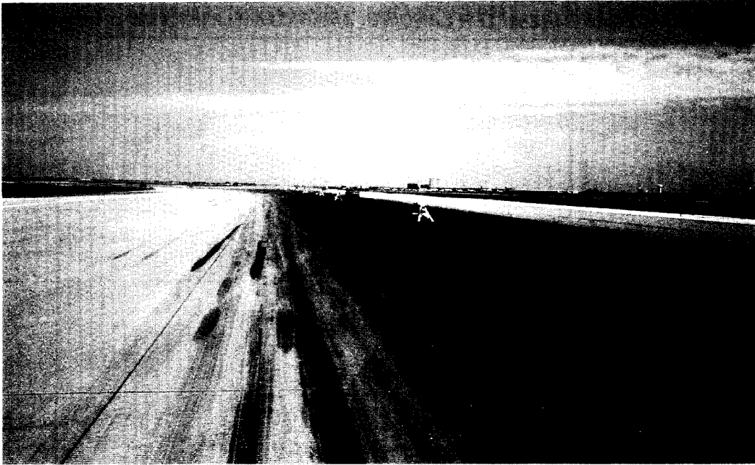
Figure 3a.--Tire marks on landing runway 17L (looking north).
