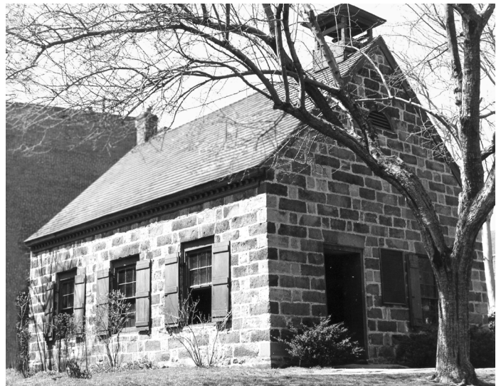
Lyons Farm Schoolhouse, ca.1782-84. Longer in proportion than the Brainerd school, its entrance was placed in the gable end, foreshadowing a change that would become standard in the 19th century.
