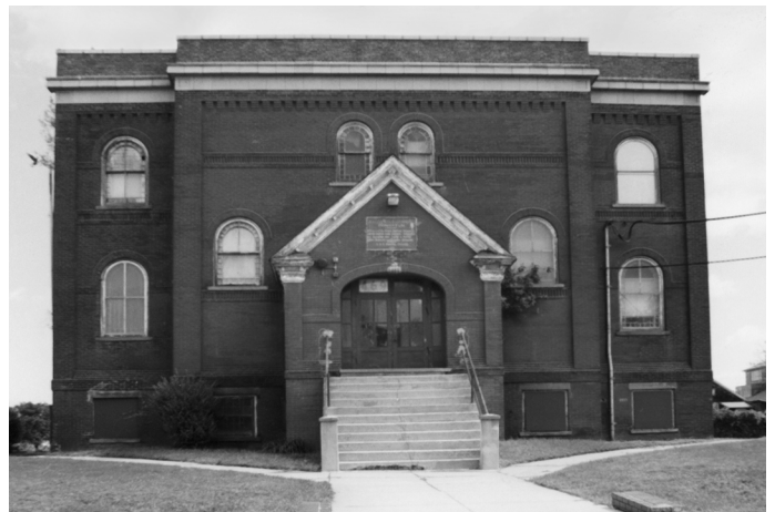
The Church Street School, Long Branch, built 1889, exemplifies two decades of schools built in New Jersey's cities in the wake of the 1867 and 1871 school laws that together ushered in the modern era of "public" education. They also served as examples for the schools built in the state's suburbs and small towns following the 1894 school consolidation act.
