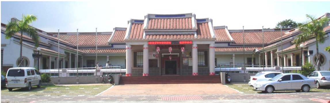
Figure 167 The prior look of the Kaohsiung Hakka Cultural Museum main mass (Taken by the author).
