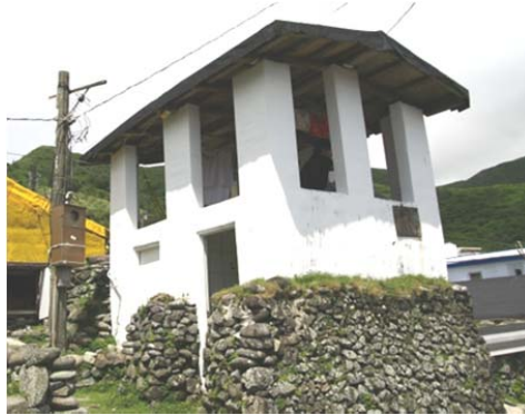
Figure 17 A traditional stilt house constructed with the modern technology in Orchid Island (Taken by the author).
