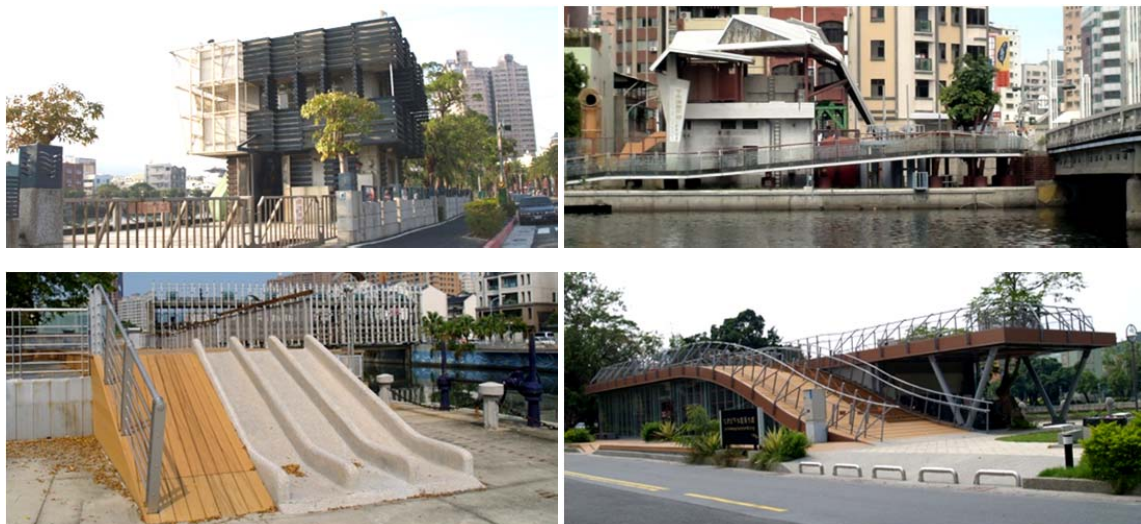
Figure 145 Four examples show the renovation result of the interceptor stations which are currently acting as Kaohsiung's urban landmarks and educational sites recording Kaohsiung's industrial past alongside Love River. The series of renovated interceptor stations is regarded as a group of cultural centres today (Taken by the author).
