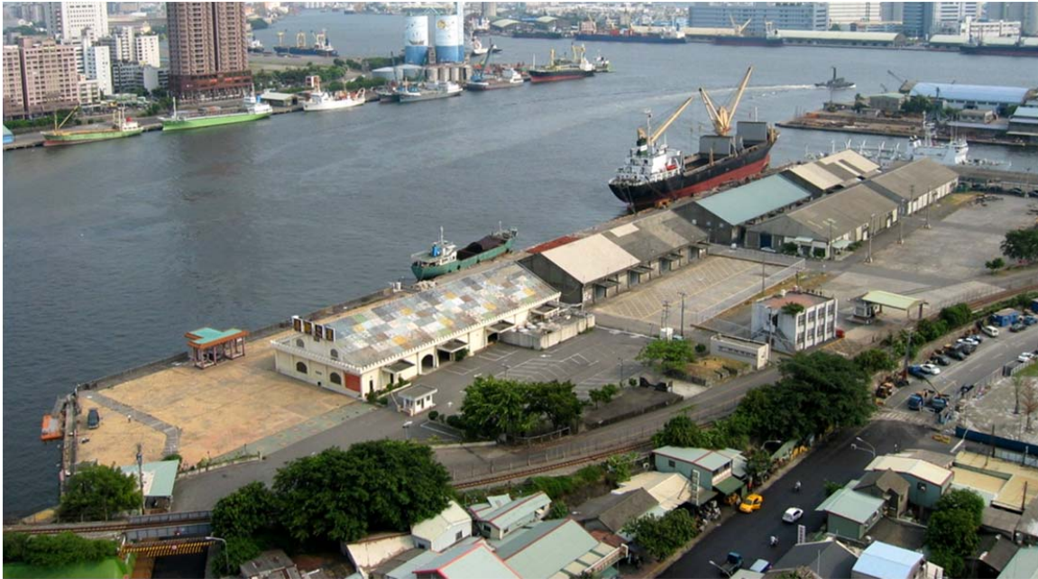
Figure 146 A prior look of Wharf 12 in the 1990s (Sourced from the Urban Development Bureau, Kaohsiung City Government).
