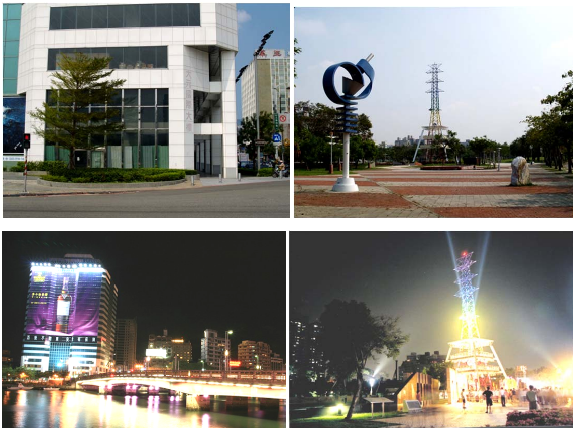
Figure 144 Two successful adaptive reuse examples in Kaohsiung's waterfront in relation to the city's recent industrialisation process by transforming once valueless sites into regional and cultural landmarks create different functions at day and night times. The left is a current unused building - Ta Yuen Building (top left), which has been renovated as an advertising and local landmark today (bottom left); the right hand pictures show an old high-voltage tower which has been renovated as an observation tower alongside Love River. These two cases are distinctive examples of revitalising disused building and former industrial symbol (Taken by the author).
