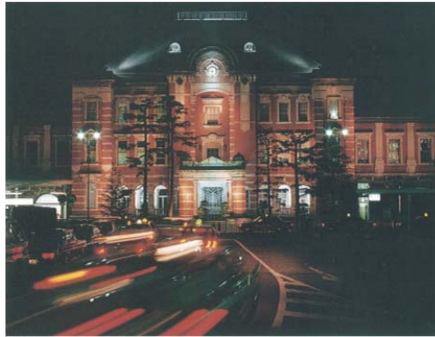
Figure 181 Main entrance of Tokyo Station (Tokyo Suteshon Gyarari, Like a Red Brick: Tokyo Station and Japanese Modern Brick Works . Tokyo: Higashinohon Ryokiyaku Tetsudo Kabushiki Kaisha, 1988: p. 37).
