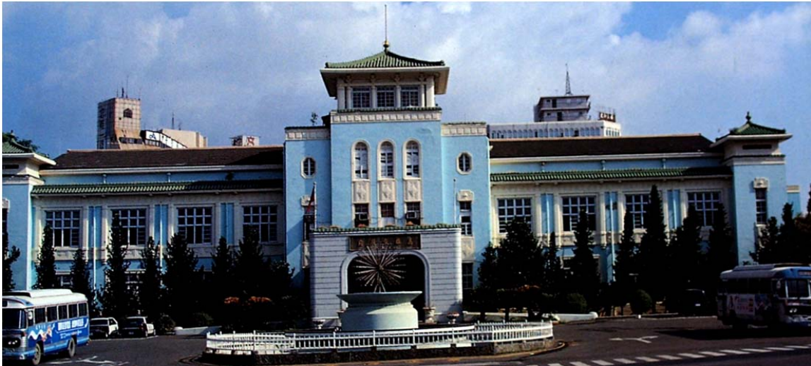
Figure 111 A picture which was taken in early post-war time still shows the defence colour - sky blue, when compared to today's grass green (Fu Chao-ching, Jih Chih Shih Chi Taiwan Chien Chu (日治時期台灣建築) (Taiwanese Architecture in the Japanese Era) . Taipei: Ta Ti Ti Li, 1999: pp. 48-49).
