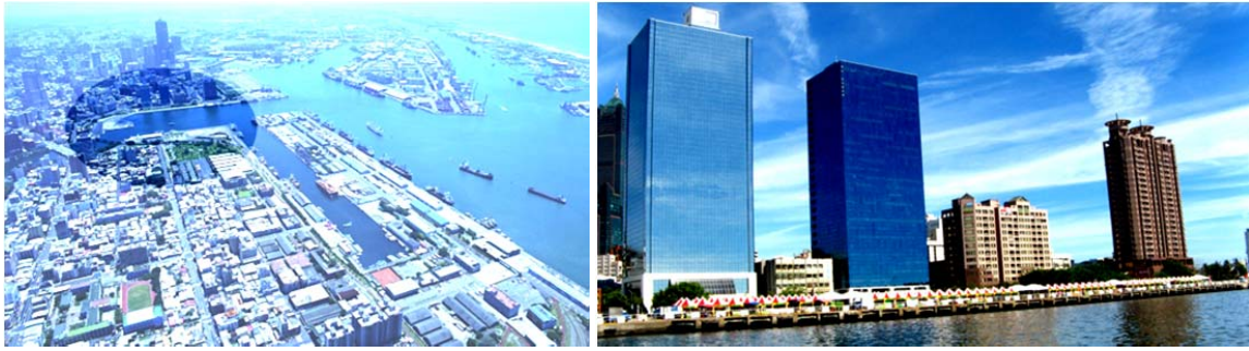
Figure 135 The left picture shows the port area of Kaohsiung. The circle in the middle indicates the area of Wharfs 11, 12 and 13 (Made by the author, sourced from the Urban Development Bureau, Kaohsiung City Government). The right picture shows the current close-to-water (water-friendly) landscape of Wharf 13 (Taken by the author).
