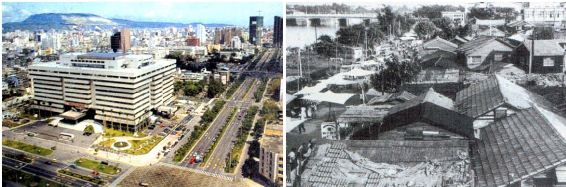
Figure 98 Two pictures show the newly constructed Kaohsiung City Hall on the current site and the simultaneous depressive situation on the neighbourhood of the old City Hall where was full of prostitutes and a lack of public security (Kaohsiung Museum of History, 2001: p. 69).
