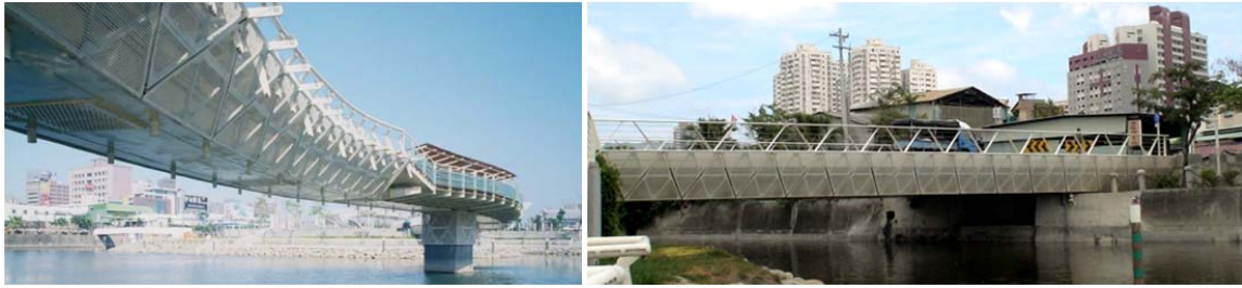
Figure 154 The left image is a bridge at the Heart of Love River; the right figure is a newly renovated bridge next to the Heart of Love River in 2010 showing a high connection to the Heart of Love River (Taken by the author).
