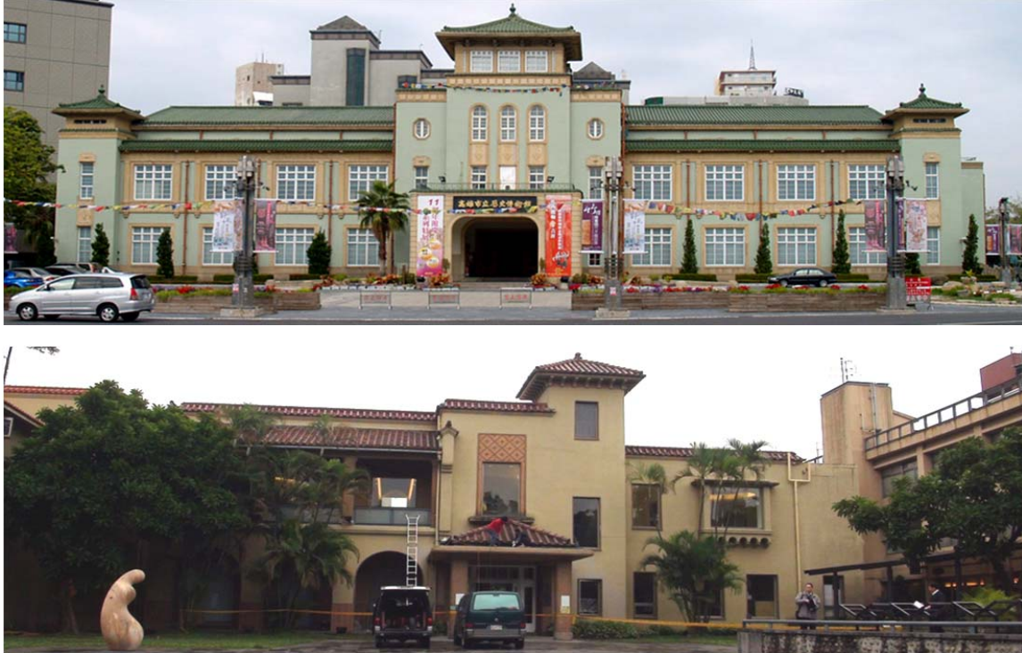
Figure 104 The upper picture is the main façade of the old City Hall building which shows a symmetric layout. The bottom picture is the main façade of the Taipei Broadcasting Bureau building which shows an organic layout (Taken by the author).
