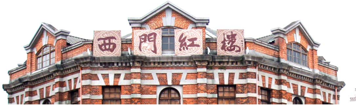
Figure 52 The pediments and dormer windows of the Octagon Building (Taken by the author).
