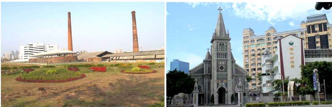
Figure 150 Two examples show the historical buildings which are integrated as elements of the group architecture in waterfront Kaohsiung being a cultural and historical indicator. The left image is the preserved former Tangrong Brick-Kiln 中都唐榮磚窯廠; the right image is the Holy Rosary Minor Basilica-Cathedral (Taken by the author).
