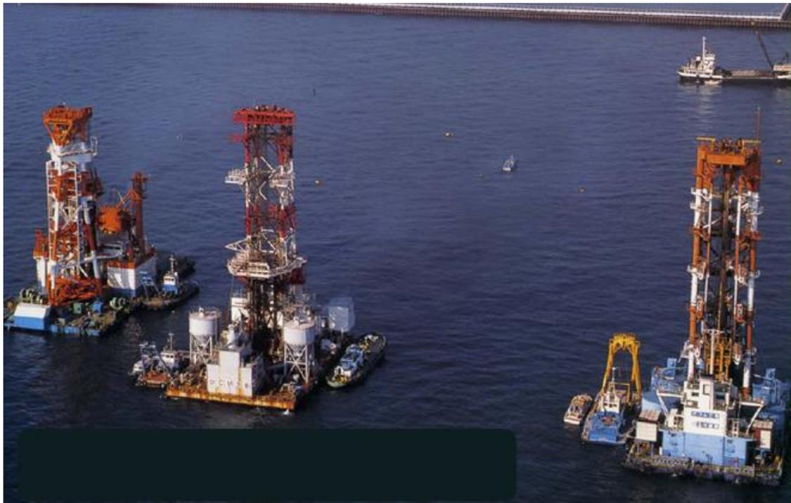
Figure 5.34 : Land Formation by Deep Cement Mixing (DCM) Method
