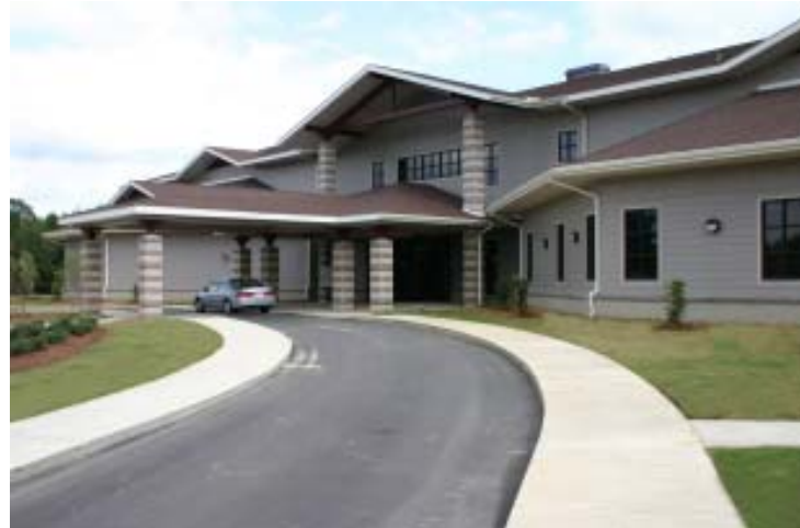
Lowery A. Woodall Advanced Technology Center
