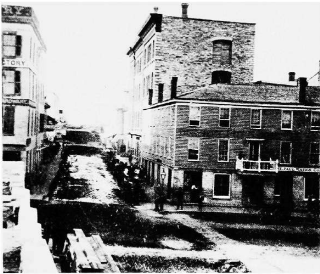
THE NEW St. Paul Water Company at Jackson and Third streets in 1869; in the left foreground, the wall of the St. Paul Fire and Marine Insurance Company, is under construction.
