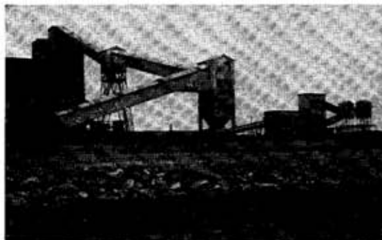
A completed steel-framed conveyor with another partly completed in the background.
