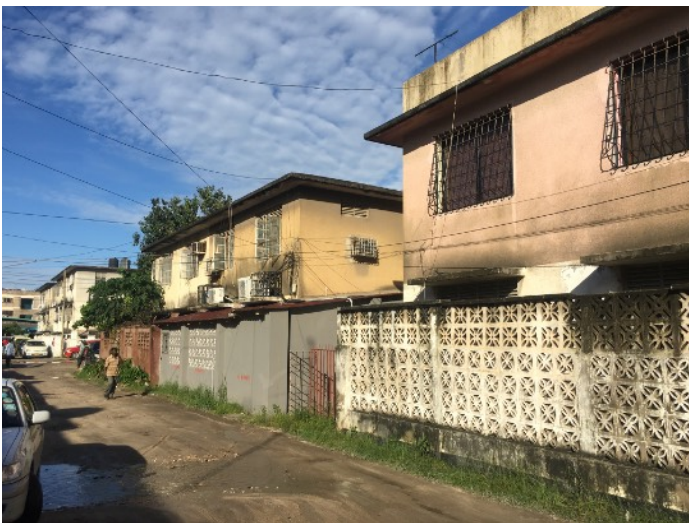
Figure 16: Neighbourhood Type 4 with walls around individual buildings.
