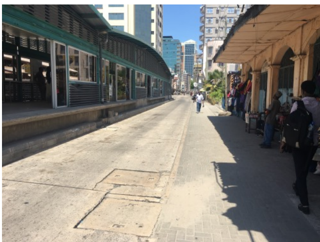
Figure 43: Narrow BRT lane and active commercial frontage at S2.
