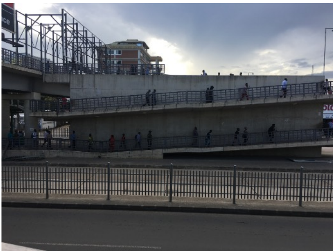
Figure 73: Ramp leading to aerial walkway for access to terminal type T2
