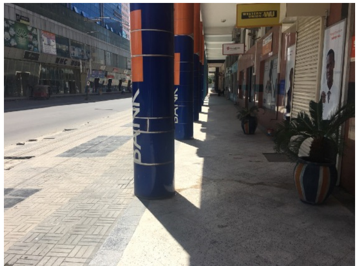
Figure 6: Sidewalks in Neighbourhood Type 1 are generally of a high quality, often embedded into the building frontage and shaded by an overhang. Most building frontages are commercially active.
