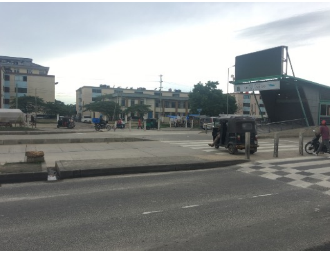
Figure 68: Station of type S7, showing connection to Neighbourhood Type 4 in the background.
