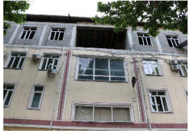
Photo 2: Front view of the Main office of MOLME
