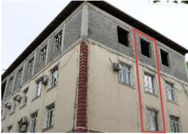
Photo 1: Side view of the Main office of MOLME, the fire ladder proposed to mount in the area shown by red
