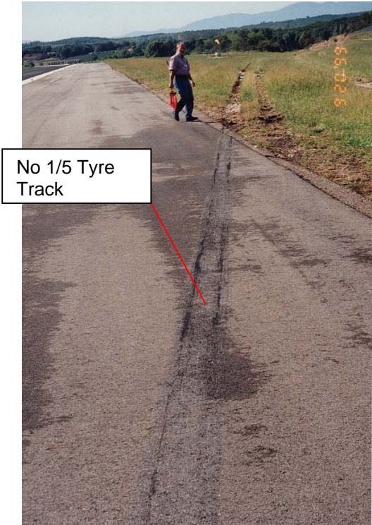
Figure 24.1 – Runway Edge Tracks
