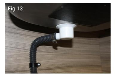
Once the water pipe is connected it should be secured to the side of the furniture approx. 200 -300mm below the tap, this is so that pressure isn't placed on the tap stem – which could result in the tap leaking. (12)
